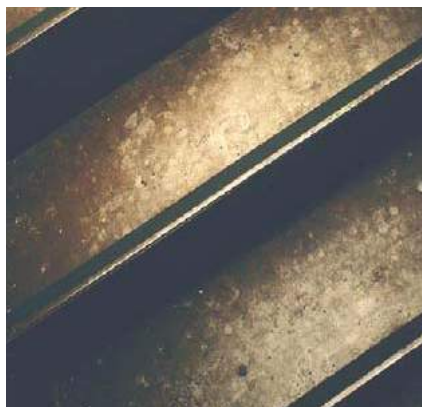
Picture 7: Anti-skid strips on the stairs
