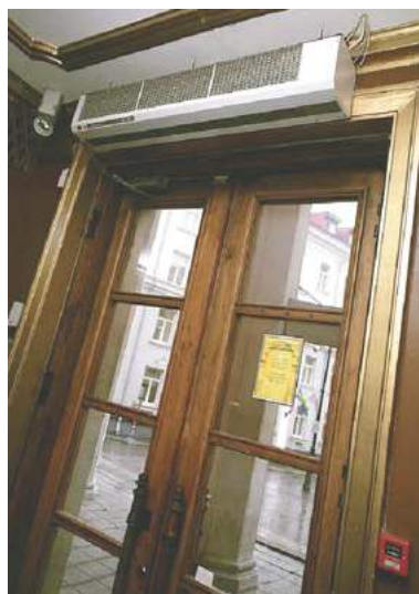
Picture 6: A blast heater at the entrance
